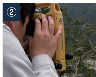
② Surveying the coordinates of GCPs
